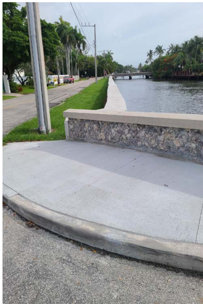
Seawalls address tidal flooding and may trap stormwater.
