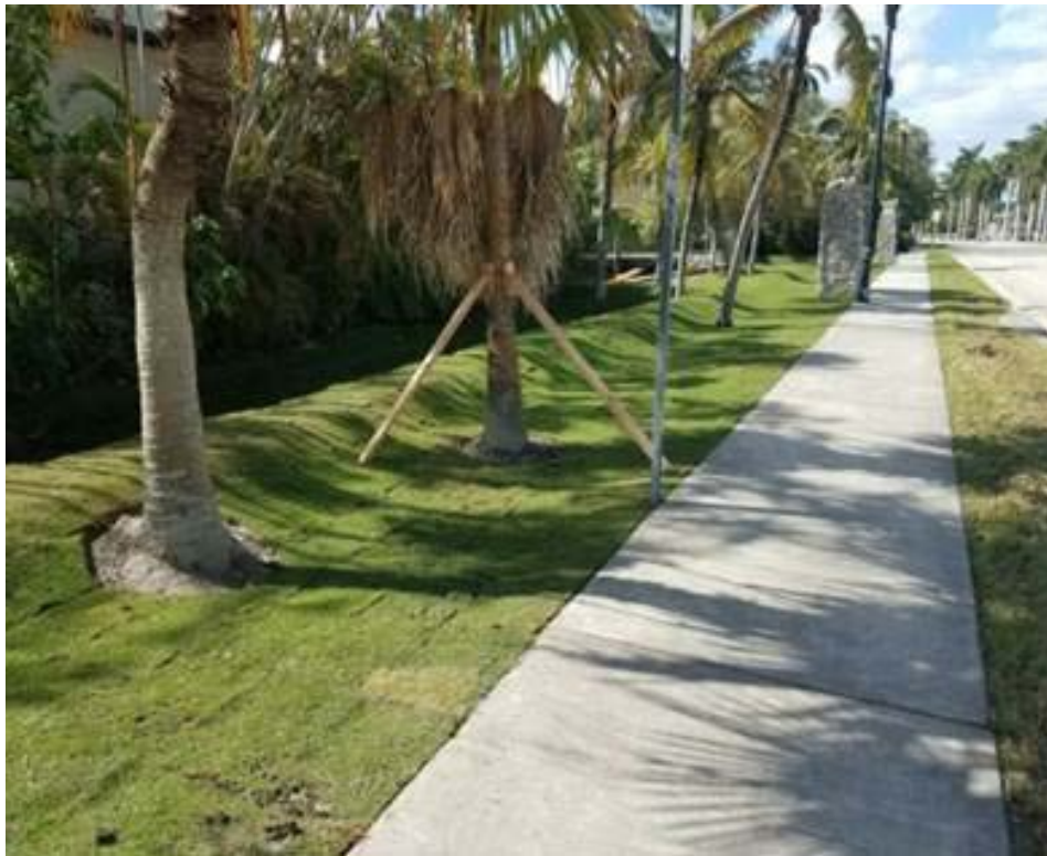
A roadside swale is an area that gently slopes to manage water runoff and can include a natural element such as grass or other pervious materials.
